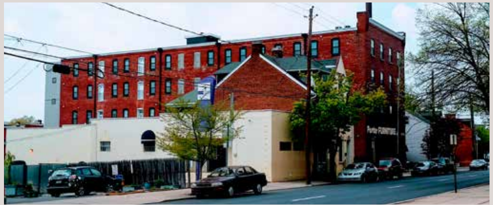
Former Porter Furniture warehouse at 626 Columbia Avenue has been converted to 24 market-rate apartments.
